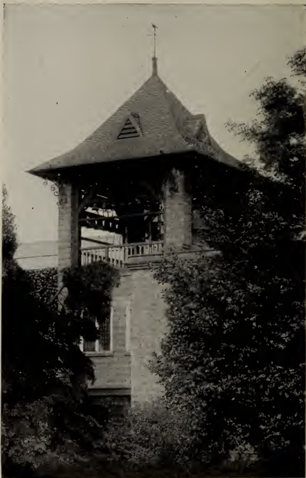
LOUGHBOROUGH: THE FOUNDRY CARILLON
